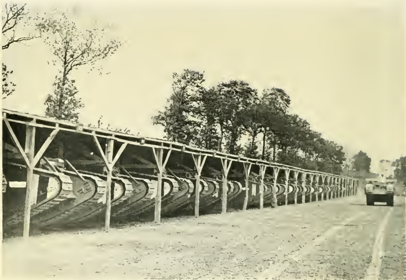
Some of the many stables where our tanks are housed. (p. 190)
